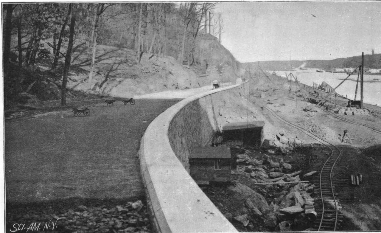
RAISED WESTERLY SIDEWALK, NORTH OF WASHINGTON BRIDGE, SHOWING RETAINING WALL, AND UNFINISHED ROADWAY AT GRADE.
