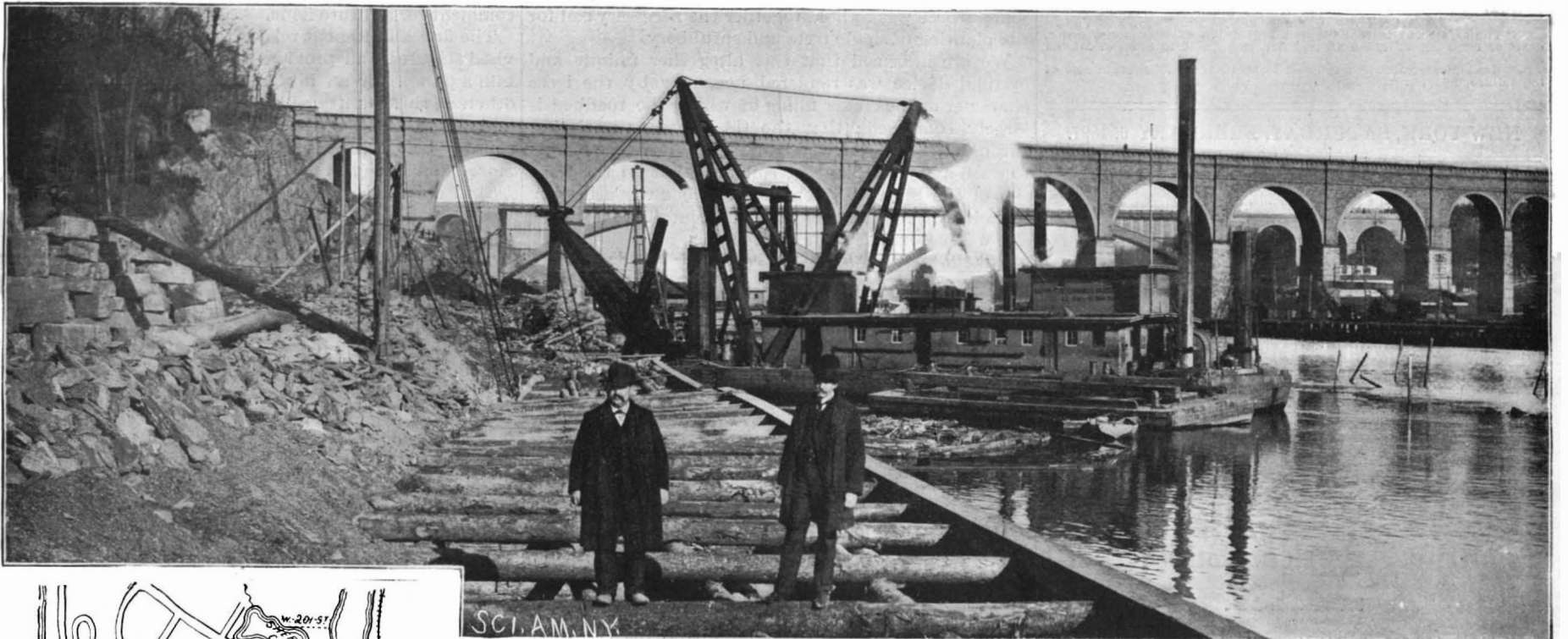
DREDGES REMOVING TIMBER CRIB, TO MAKE WAY FOR MASONRY CONSTRUCTION.
