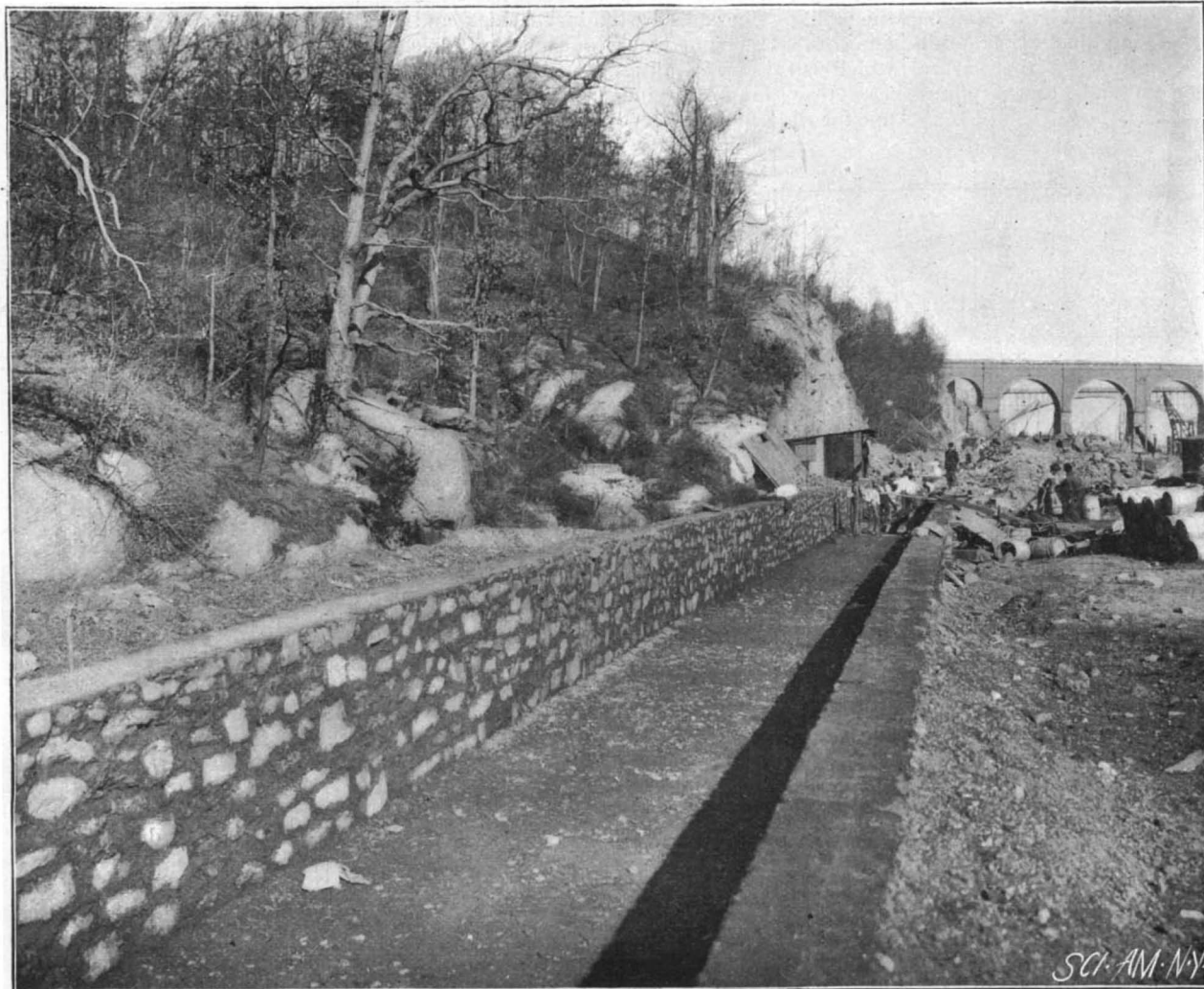
HARLEM RIVER SPEEDWAY—UNFINISHED ROADWAY SOUTH OF HIGH BRIDGE, SHOWING SOLID MASONRY TRENCHES IN WHICH TO PLANT SHADE TREES.
