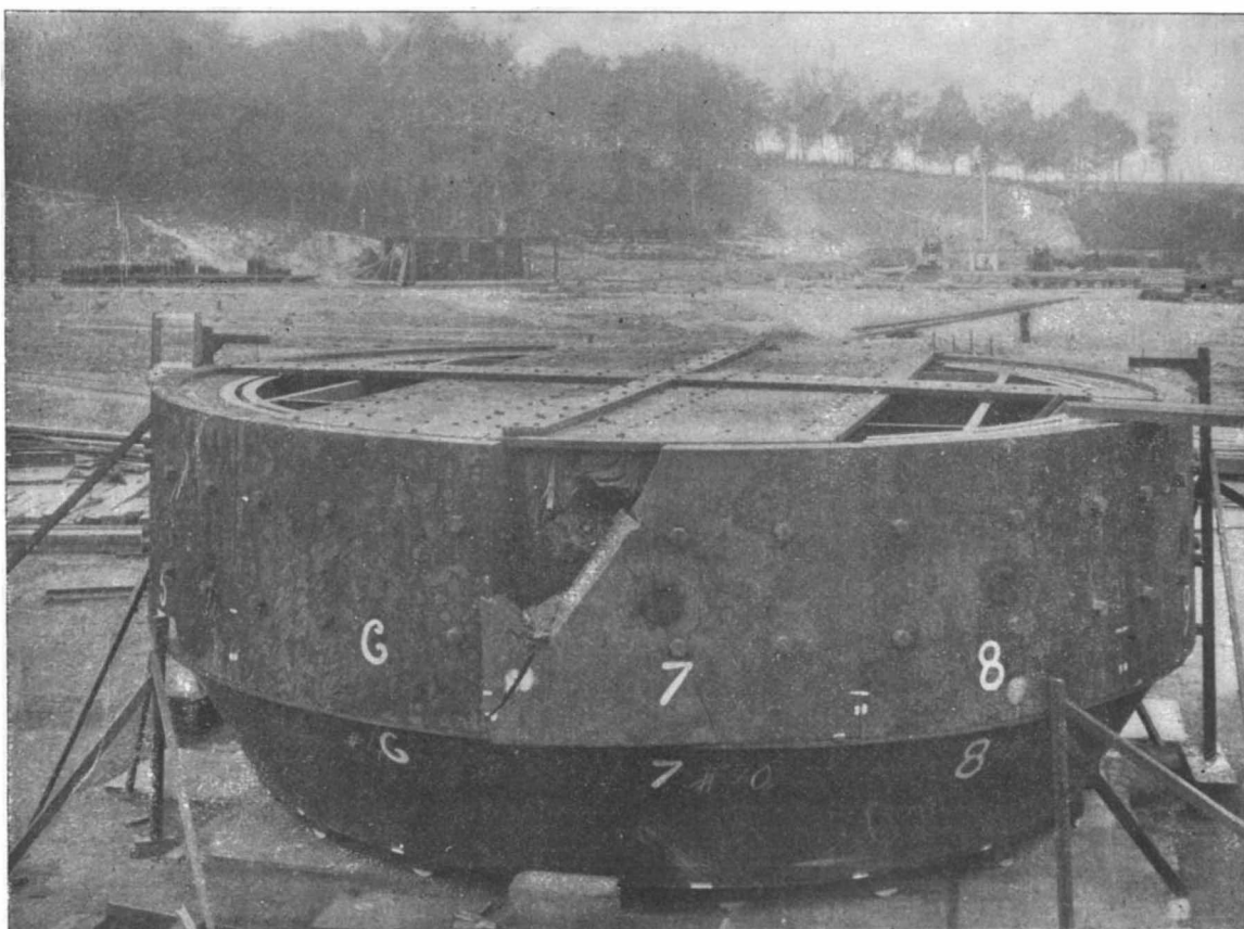
EXTERNAL VIEW OF REAR WALL, SHOWING DESTRUCTION OF 15 INCH PLATE BY FRAGMENT OF SHOT WHICH PASSED THROUGH TURRET. 12 INCH GUN SHOWN IN THE DISTANCE.
