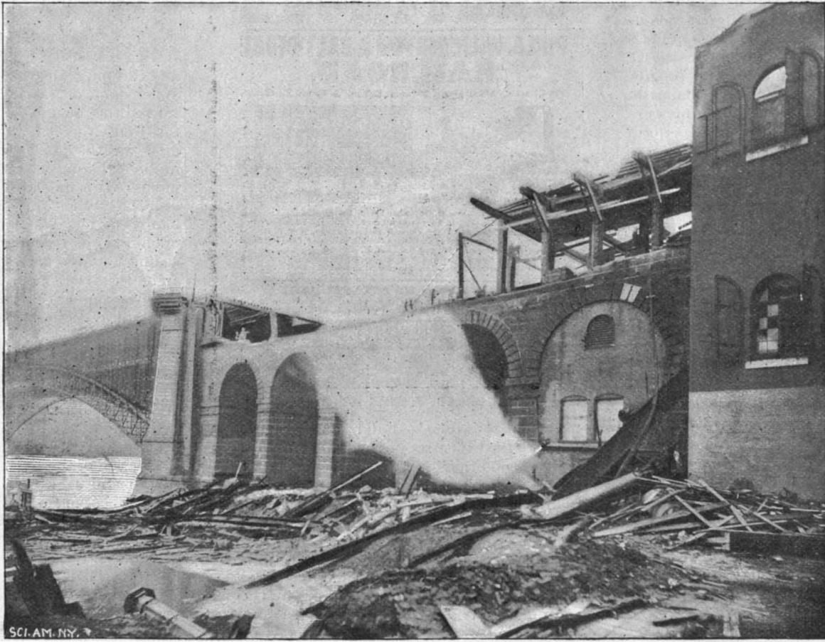
THE ST. LOUIS BRIDGE AFTER THE GREAT STORM OF MAY 27, SHOWING INJURY TO STONE WORK ONLY.
