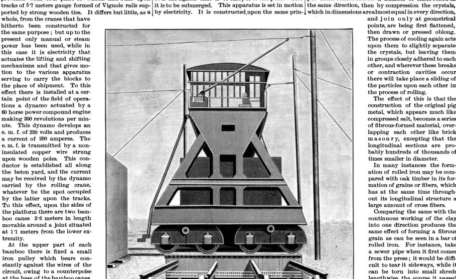
Fig. 3.-SIDE VIEW OF THE LIFTING APPARATUS.
