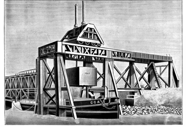
Fig. 1.-WORK AT THE PORT OF BILBAO-FRAMEWORK AND APPARATUS FOR LIFTING BLOCKS OF BETON AND LOADING THEM ON A BARGE.
