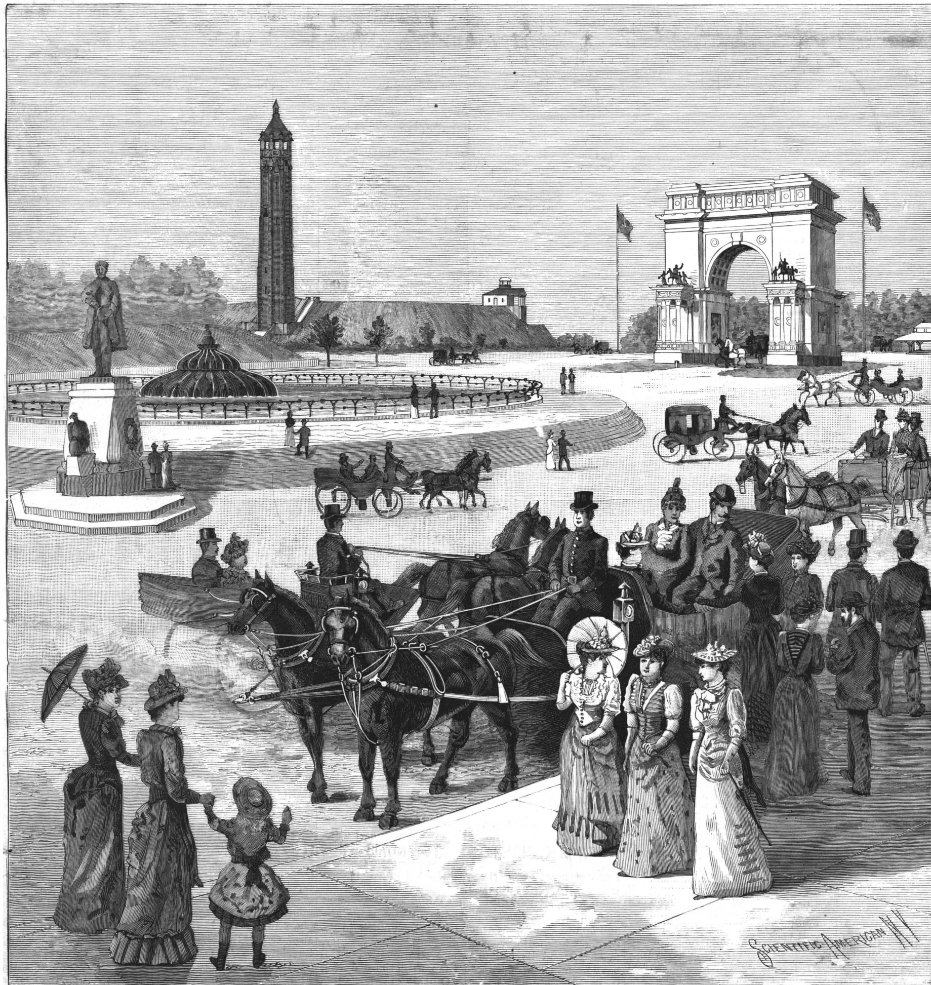
THE NEW HIGH-SERVICE WATER TOWER, BROOKLYN, N. Y., AND PROSPECT PARK PLAZA.
