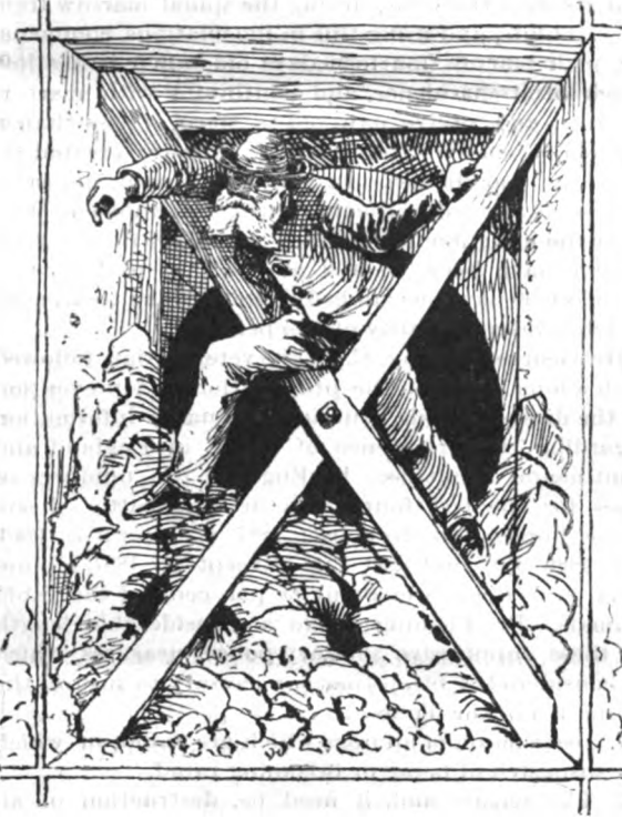
CHIEF ENGINEER HOBSON BREAKING THROUGH FROM CANADA TO THE UNITED STATES UNDER THE ST. CLAIR RIVER.
