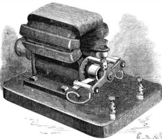
HALL'S ELECTROPLATING DYNAMO.
