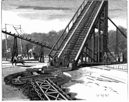
THE RELOADER SHOWING METHOD OF RAISING AND DELIVERING COAL INTO THE BARGE.
