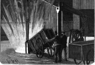
Fig. 3. TALLAPOOSA BLAST FURNACE-CHARGING THE FURNACE.
