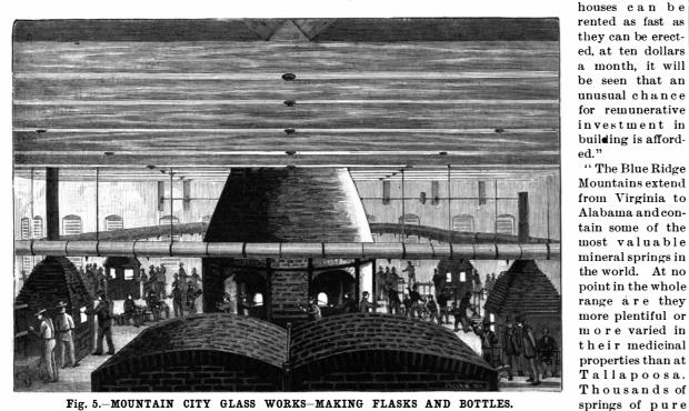
Fig. 5.-MOUNTAIN CITY GLASS WORKS-MAKING FLASKS AND BOTTLES.
