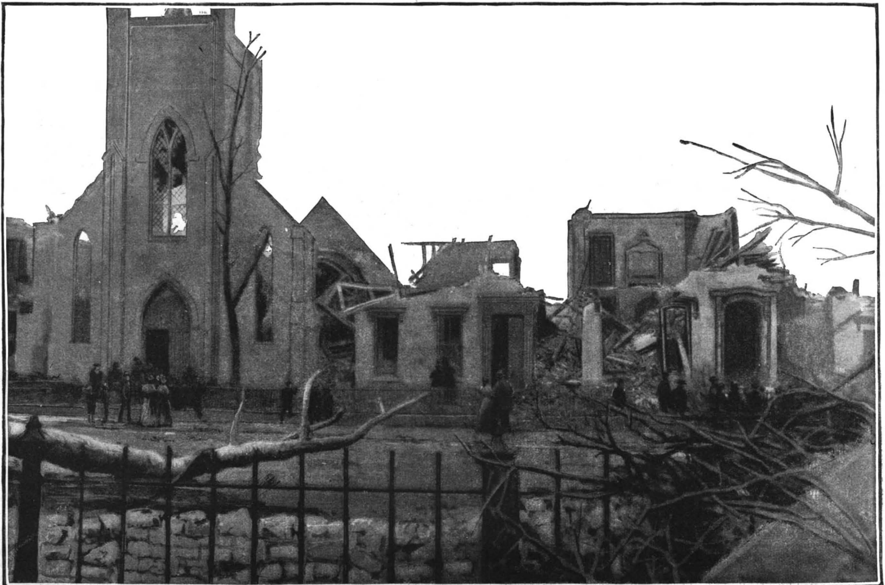
DESTRUCTION AT ST. JOHN'S EPISCOPAL CHURCH, FRONTING BAXTER PARK. —(From a Photograph by Elrod.)
