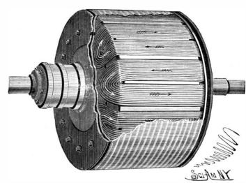
Fig. 5.-ARMATURE OF DYNAMO.
