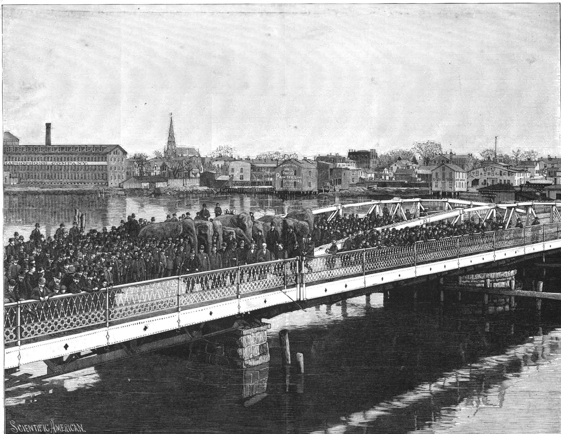
TEST OF A NEW BRIDGE BY MEANS OF ELEPHANTS, AT BRIDGEPORT, CONN.
