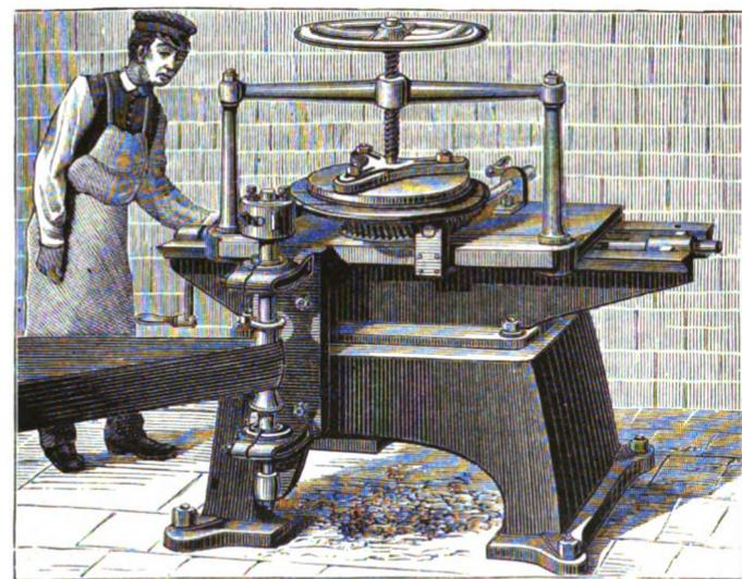
Fig. 4.—MACHINE FOR TURNING AND CHAMFERING BARREL HEADS.
