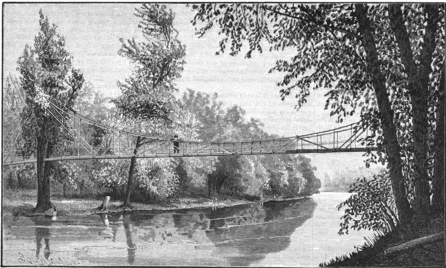
A CURIOUS SUSPENSION BRIDGE NEAR CHICAGO, ILL.
