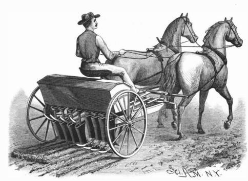
MITCHELL'S CLEARING ATTACHMENT FOR GRAIN DRILLS.
