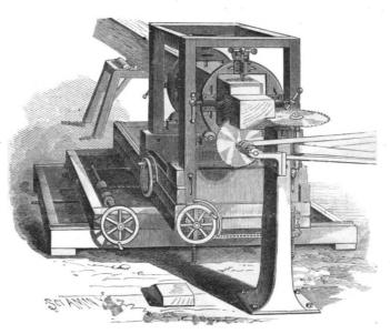
BLEY'S MACHINE FOR FRAMING TIMBER.
