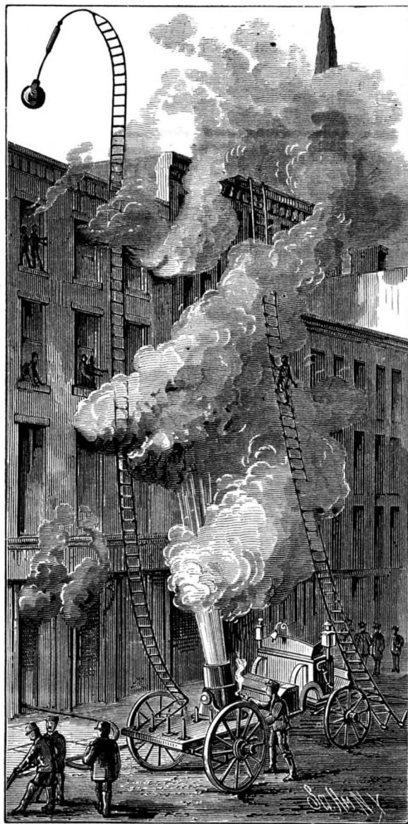
WATTS' FIRE ESCAPE.
