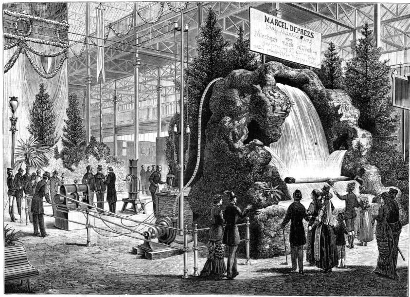
DEPREZ'S EXPERIMENT ON THE TRANSMISSION OF POWER FROM A DISTANCE BY ELECTRICITY.
