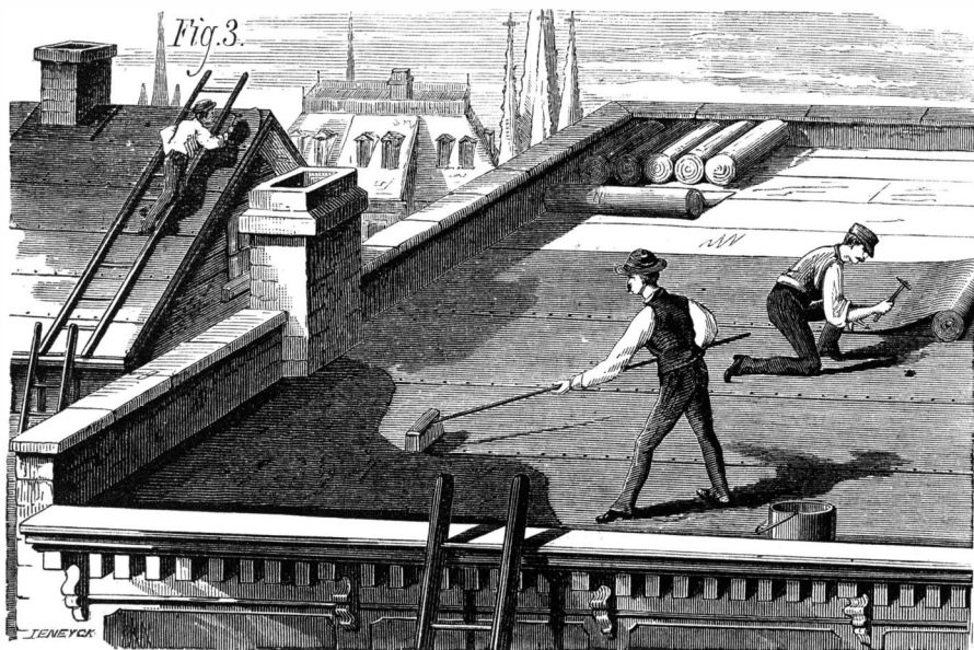
LAYING DOWN ASBESTOS ROOFING.
