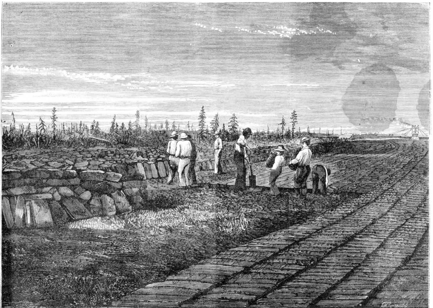
PEAT FUEL MANUFACTURE IN CANADA.—DRYING AND STACKING. (See page 356.)
