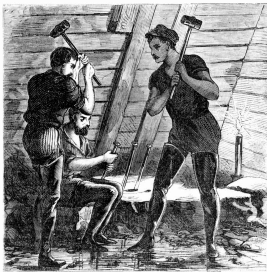
4.—DRILLING THE ROCK AT THE SHOE OF THE CAISSON.
