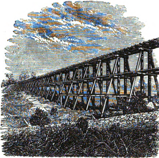
No. I.—TRESTLE OPPOSITE AUBURN.
