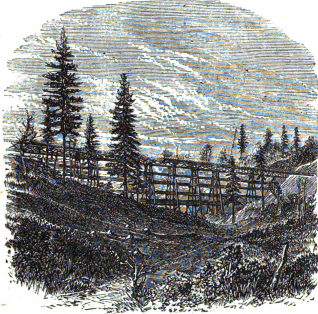
No. II.—TRESTLE AND TRUSS BRIDGE, CLIPPER RAVINE, 100 feet high.
