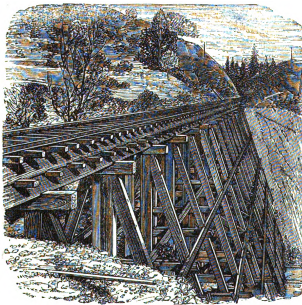
No. VI.—FIRST TRESTLE IN CLIPPER RAVINE.
