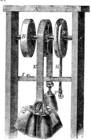
A three-ply belt of the same diameter, length, and thickness as the leather one, was chosen, and being loaded with 32 pounds to keep it "taut," weights were added, as in the former instance, and the result was as follows :---
