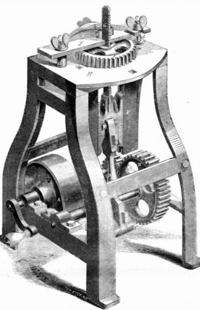
ecured to it by clamps passing through the i tightened by a screw, a. This is a remarkatable itself, as well as by a permanent clamp, J, that is held down on the wheel by the screws, d, and nuts, c. The saw, G, works up and down in a slot in J, and it is pressed against the inner periphery, or provided with | further particulars upon being addressed as the requisite feed by a spring, a, that can be above.
