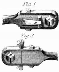
ward underneath the seat, D, as is also indi- | interfere with the graceful appearance of the cated by dotted lines. so that by moving D forward when there are two seats, only one seat will be obtained, and when there is only one seat, moving D backward will bring out C, making two seats. The seat, C, may be made to form a box for containing any necessary accompaniments to a vehicle, and this method of constructing buggies does in no way
