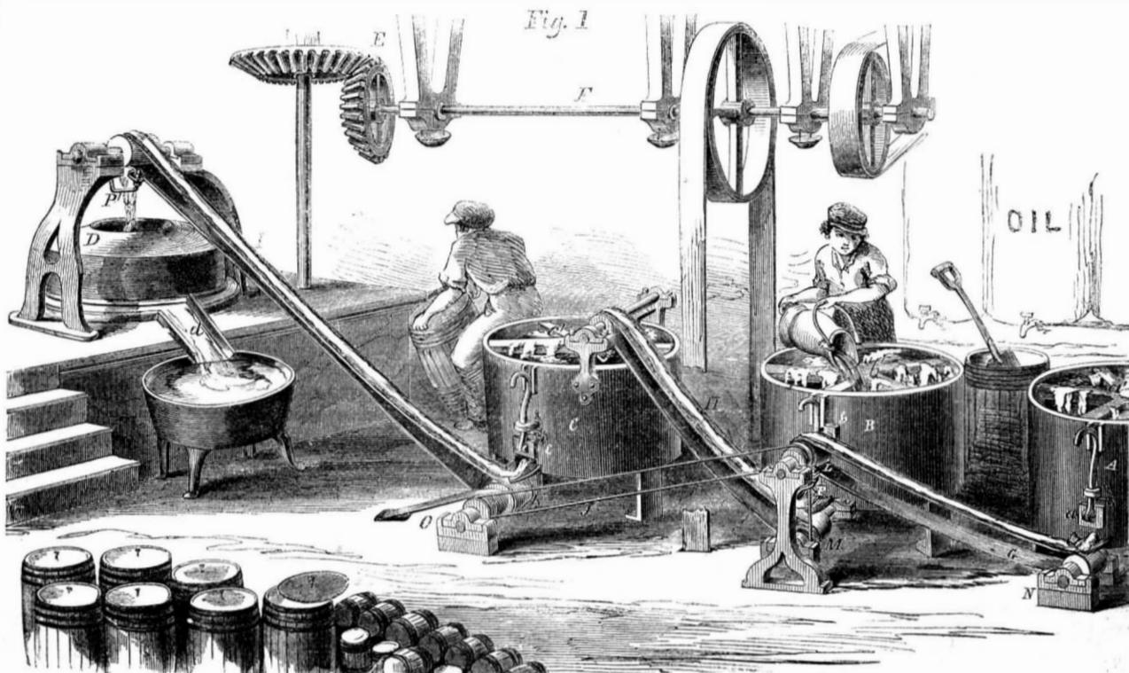
In the mixing of white lead and other paints, there are many difficulties to encounter, one of the greatest being in feeding the millstones regularly and constantly, so that an even and smooth paint may be obtained.
