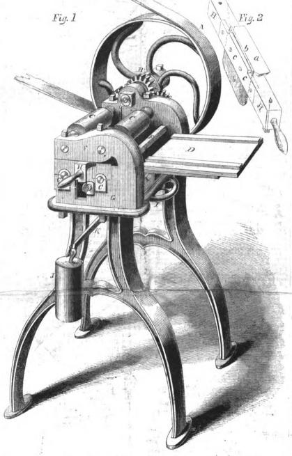
calls it, "a machine for smoothing wood arfaces," is quite unlike any of the ordinry smooth wood from one-thirty-second of in inch thick up to almost any size desired. It word, but slices off the shavings, and will o quality in the surface of the wood. slice them until the plank or other piecof wood is perfectly smooth.
