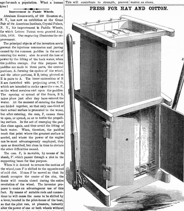
Cotton and Hay Press. sists in its simplicity, cheapness or construc Our engraving is taken from a full-sized tion, durability and great power. The sub-Press now on exhibition at the Crystal Pal- stance to be pressed is placed between the than the other, and that the vessel may be ace. The chief merit of the improvement con- follower, A, and bottom board, B. The pres
